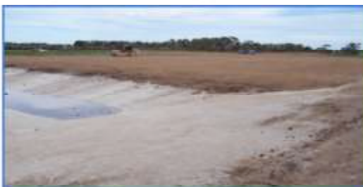
Abattoir waste composting site & holding dam
