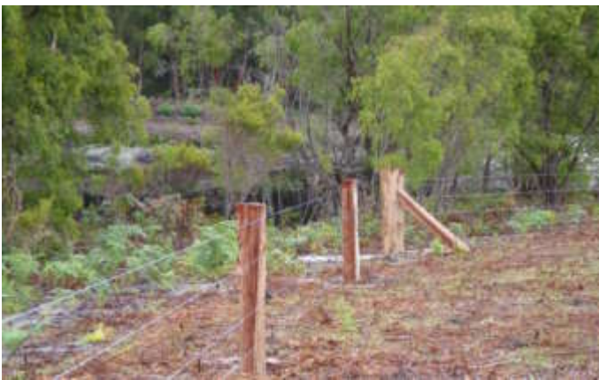
Newly completed waterway fencing
